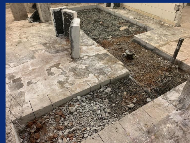
Saw Cutting of Slab in Area H.
