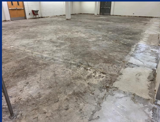
Demolition of Floors in Area H
